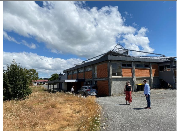
Photograph 3: 29 Hamilton Street, looking northwest
