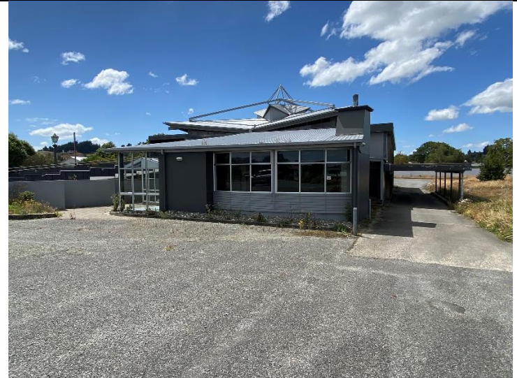
Photograph 2: 29 Hamilton Street, looking east across the carpark.
