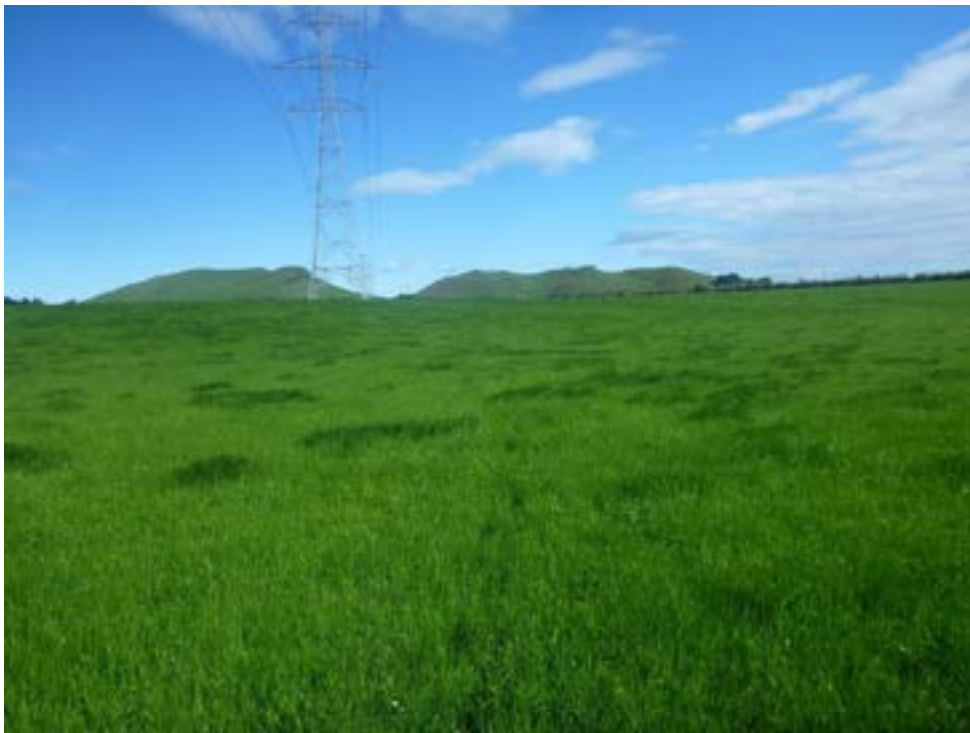
Figure 4: Existing power pylon within the proposed transmission extension envelope, November 2023.
