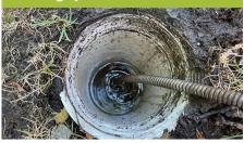
This is a cleaning eye, or access point, that's an important part of your domestic wastewater drain. Sometimes it gets lost over time. It may be overgrown, it may be under paving, or it may simply be overlooked.
