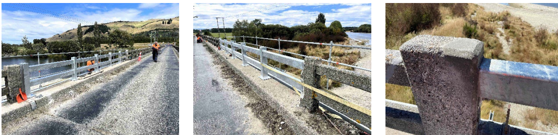
Otamita Bridge handrail repair close to completion
