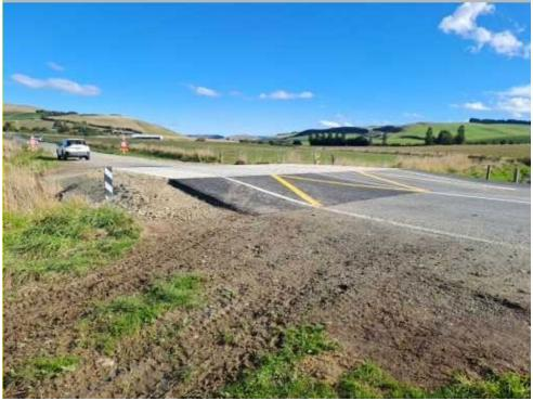
Waikana Road Armco culvert bridging
