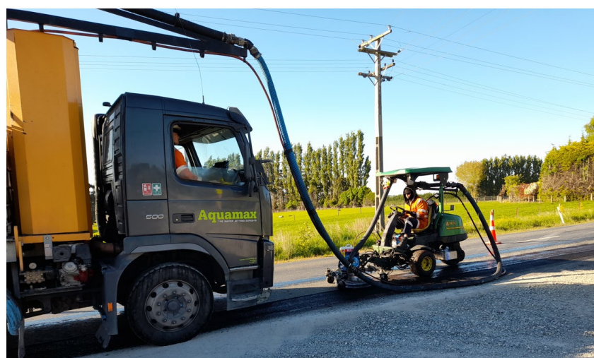
Watercutting excess bitumen from sealed pavement – Reaby Road
