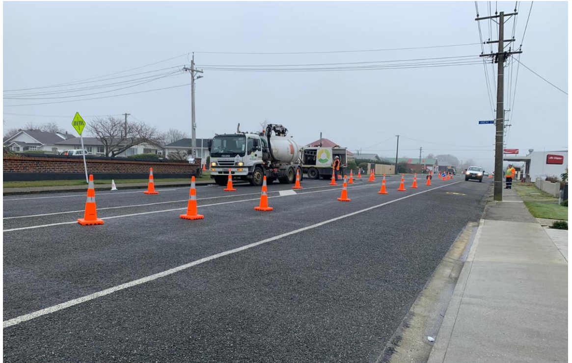
Photo 1 – The Council's contractor cleaning the wastewater main on Anzac Street in preparation for CCTV inspection
