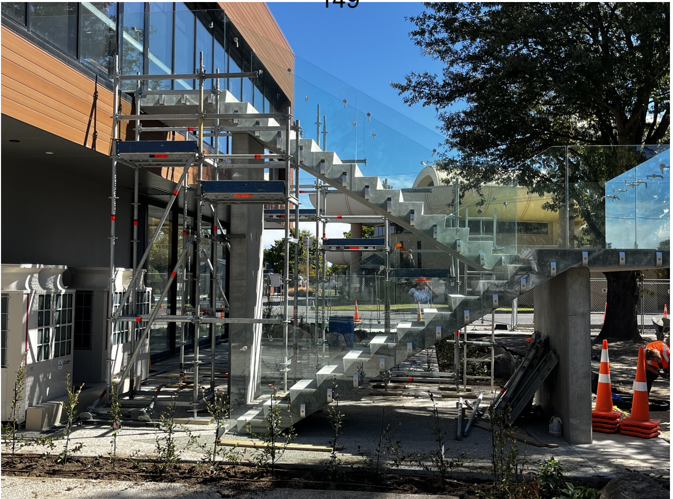
Exterior Stair with glazing in progress
