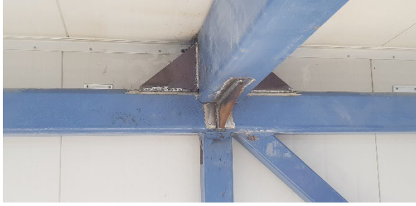
Strength welds on truss and beams
