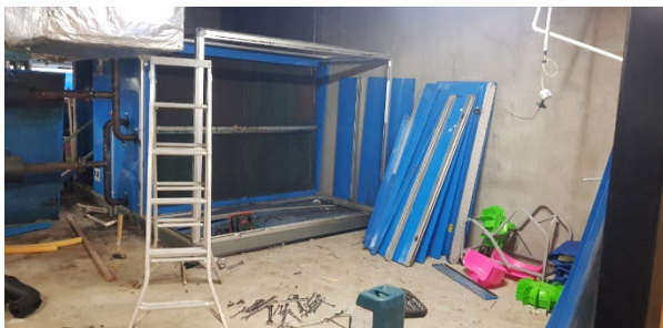
Old ventilation being removed
