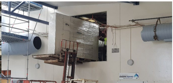
New power board going into upper plant
