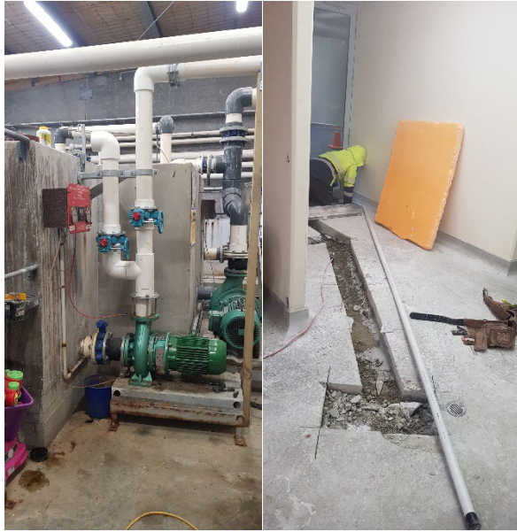
New filter pipe work
