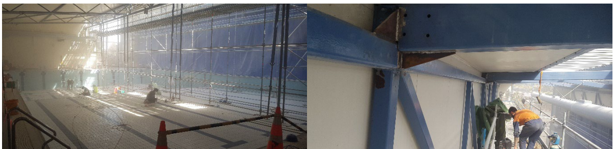
De-grouting of main pool
