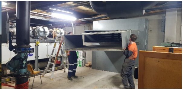
Old ventilation being removed
