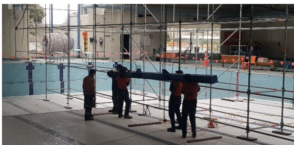
Supporting beam for new ventilation
