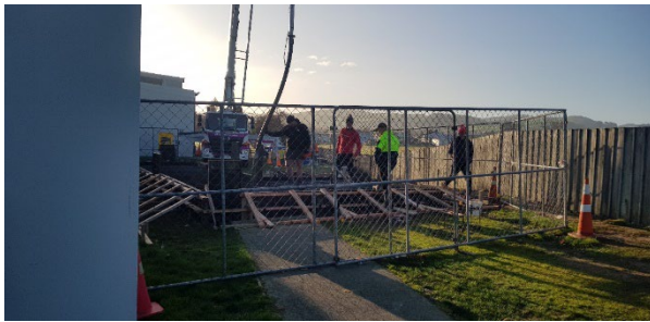
Concrete pad being poured for ventilation
