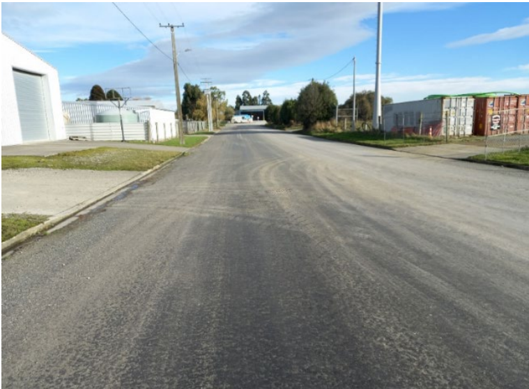
Photo 3 – Sediment build up along Aparima Street
