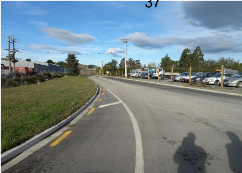
Photo 4 – Sediment build up along Falconer Road
