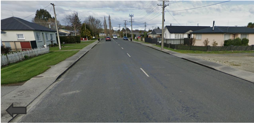
Figure 2: Hamilton Street (Outside the Site looking South)
