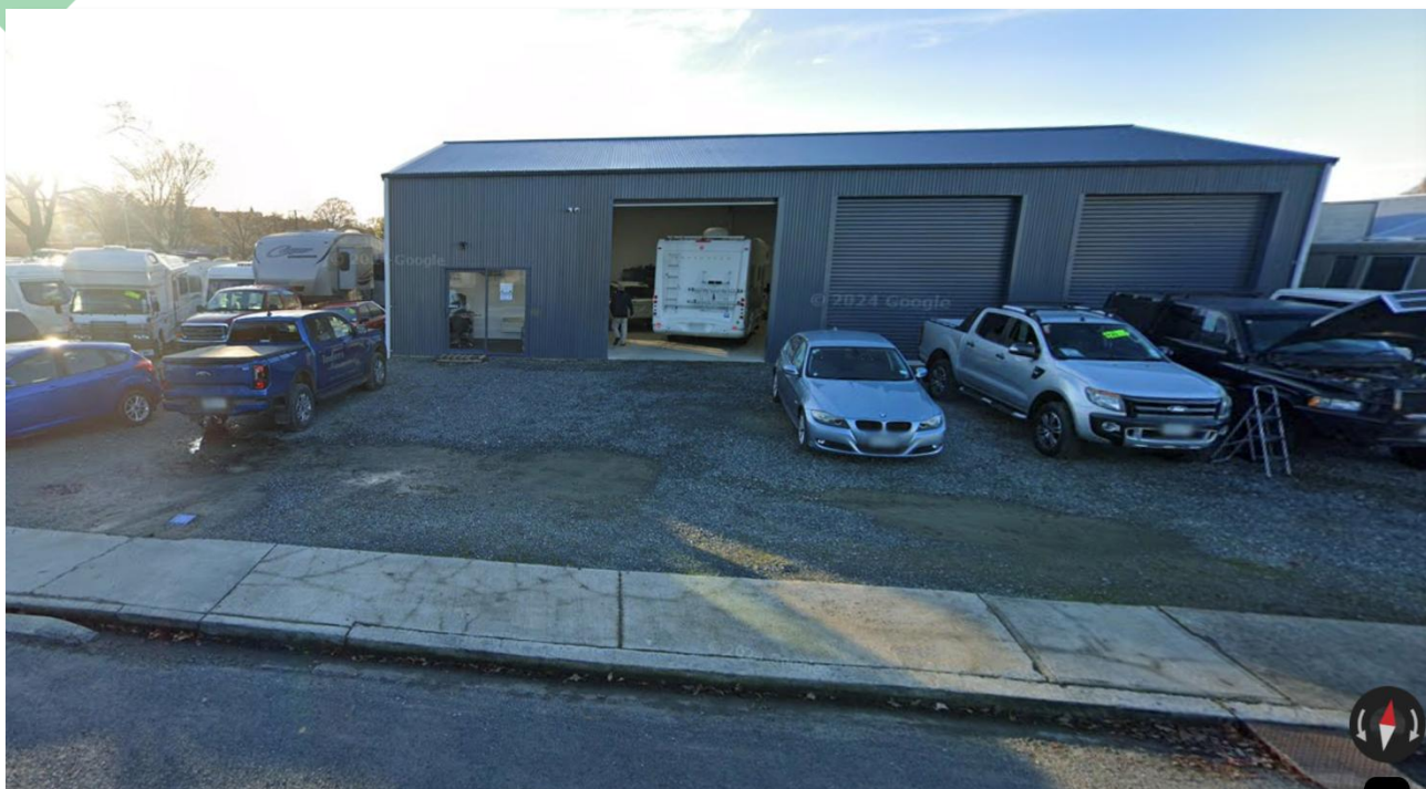
Figure 3 – South side of site, 2 Avon Street showing roller doors & site entry
