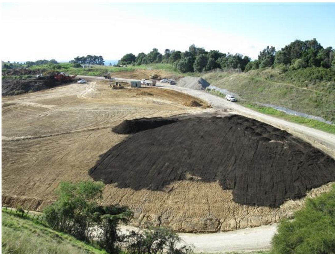
Photo 1: Spreading green waste mulch on the clay capping at Burma Road landfill 2011. Batter on front face is 3;1.
