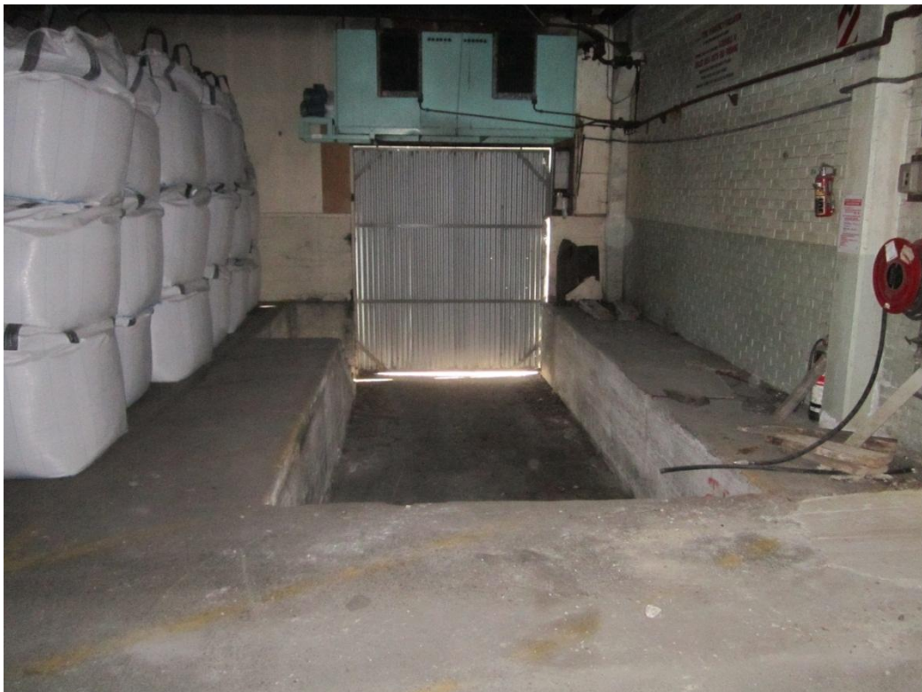
Figure 7: Sandbagging the entranceway will create a suitable location for the capture of contaminated water following a flood
