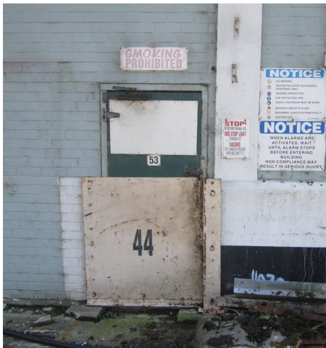
Figure 4: Example of purpose built barriers that could increase the protection to 109 Kana Street
