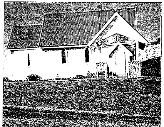
(g) The completed Lychgate in front of the former Mandeville Anglican Church.
