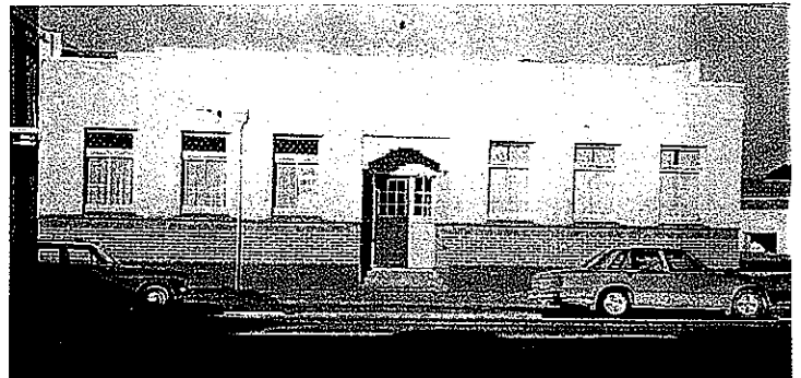
(c) The Rest Rooms building was located immediately north of the Railway Station.
