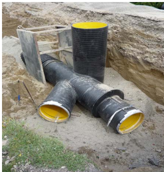
Salford Street sewer
