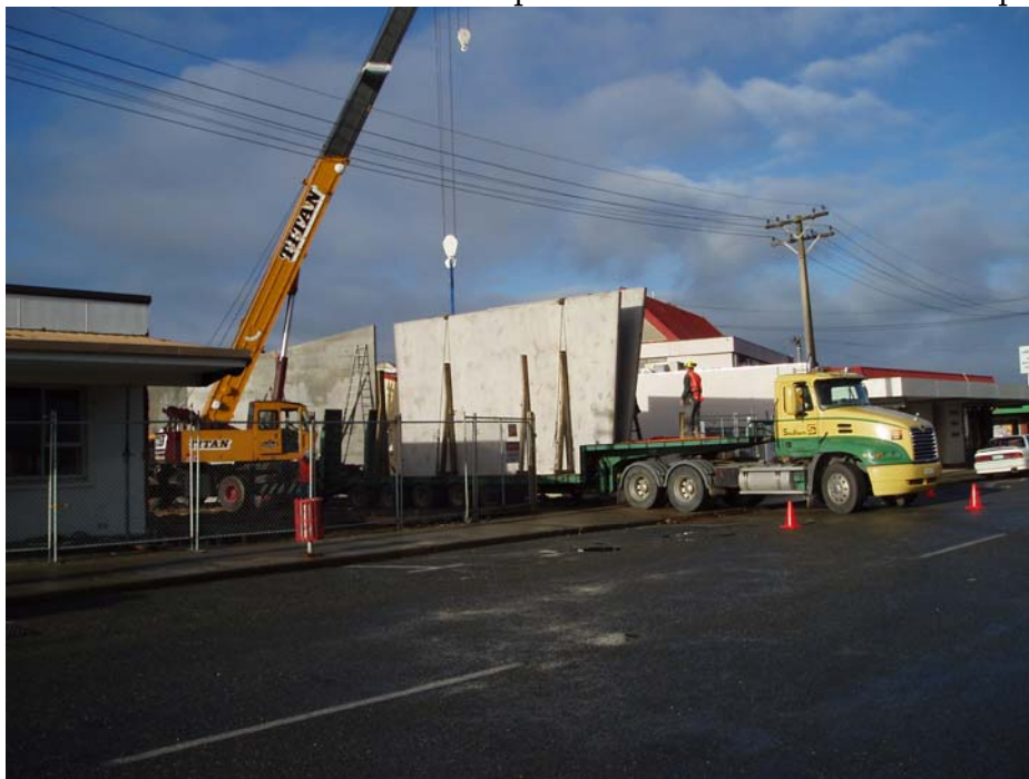
Pre-cast concrete slabs being delivered and placed onsite.
