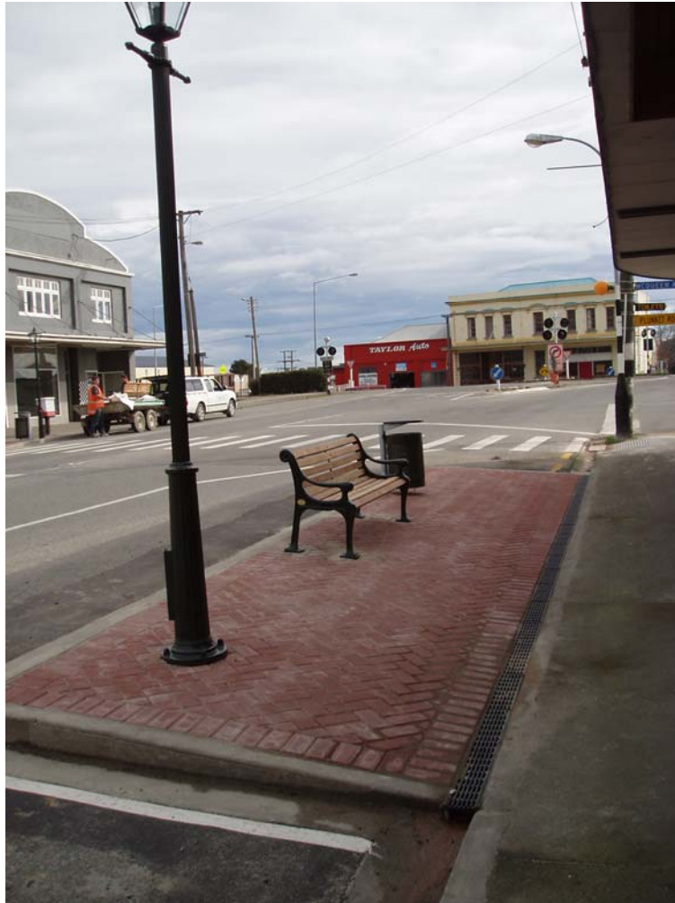
Newly developed area outside the Maitava Service centre
